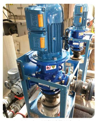
Installation of two INNOMAG TB-MAG sealless pumps with custom vertical mounting
