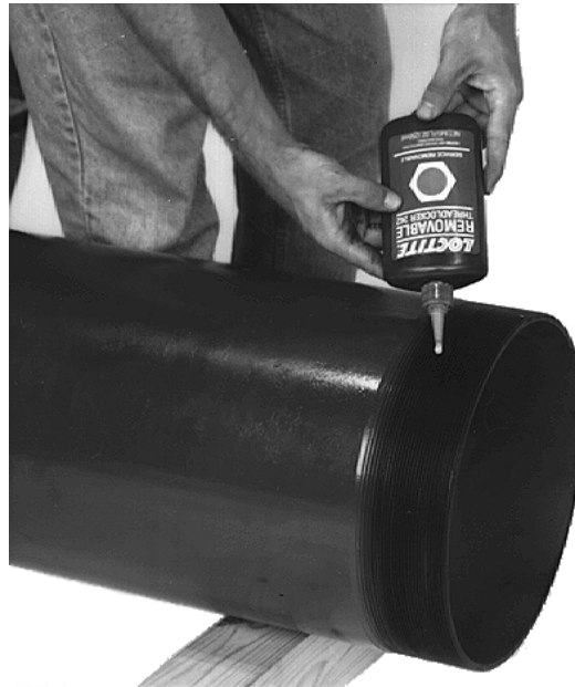
Fig 5.2.10a Cleaning threaded column pipe threads
