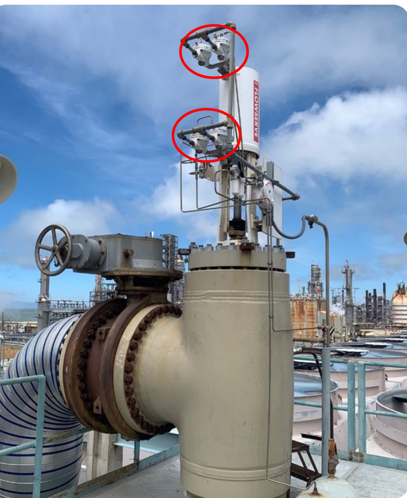
Figure 1: To achieve fast stroke speeds and precision control, plants have used increasingly complex arrangements of volume boosters (circled).
