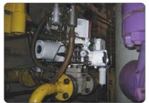
StarPac® intelligent control valve installed in the Monopod well room Photo courtesy Flowserve Corp.
