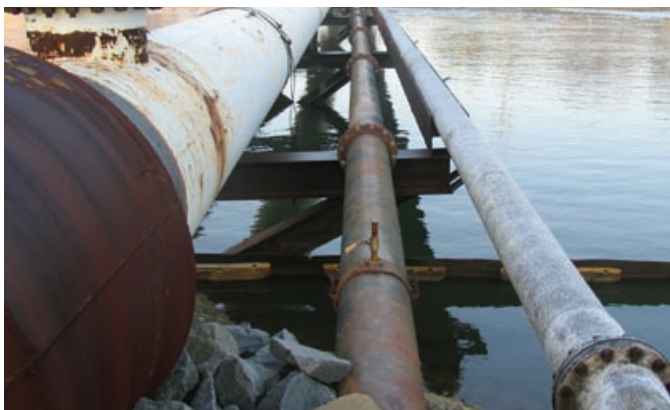
Section of existing header piping to be upgraded to larger diameter
